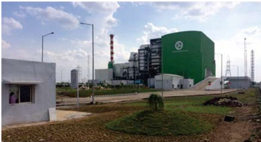
Jabalpur Waste-to-Energy Plant on PPP mode
